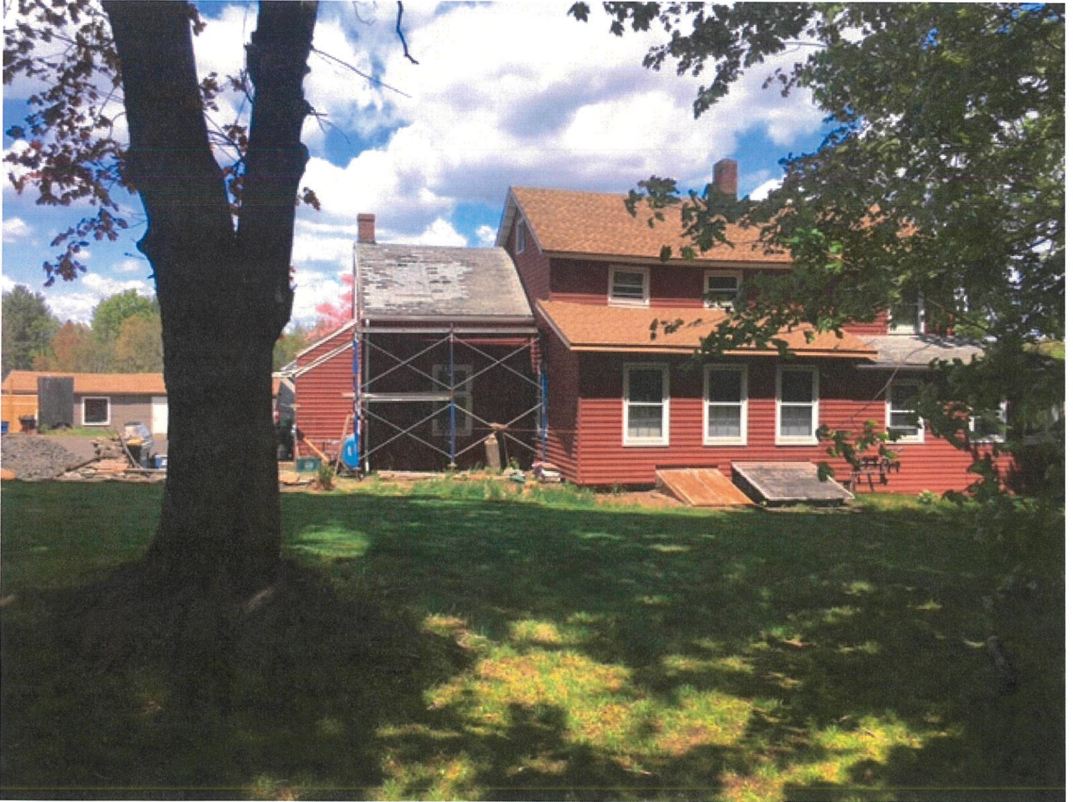
Blight 1 Bassett Road 05-12-2021
